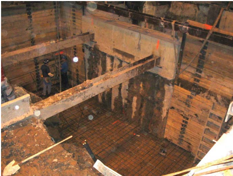
Figure 9: Completed secant pile wall and bracing
