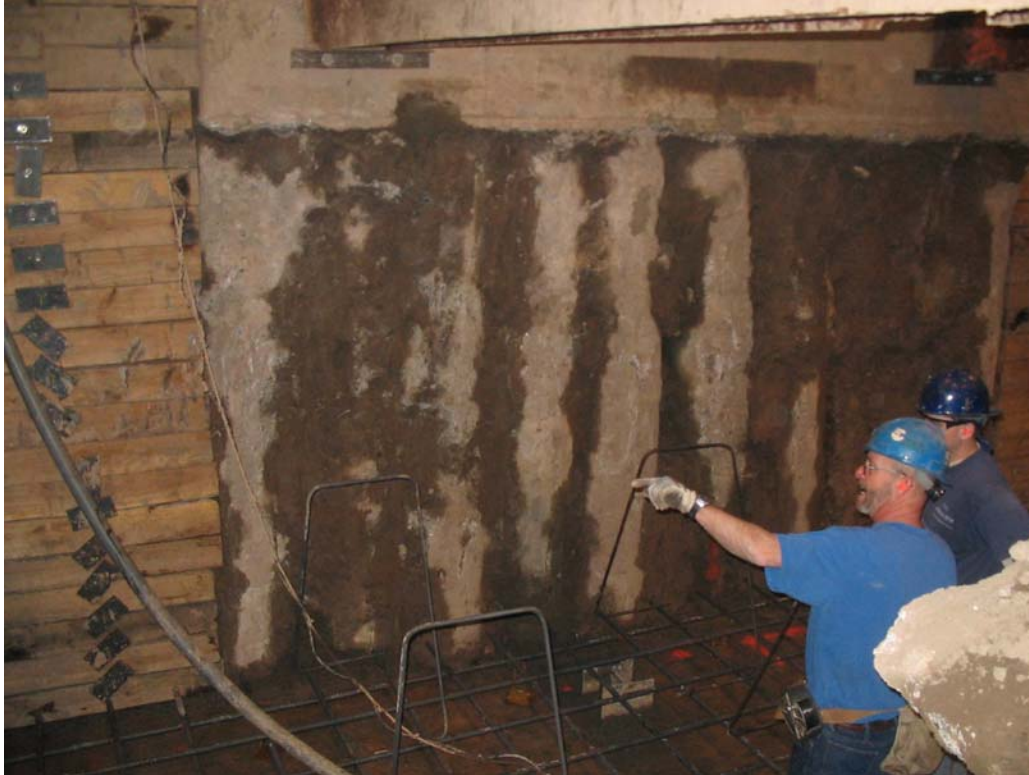
Figure 10: Close up view of completed secant pile wall
