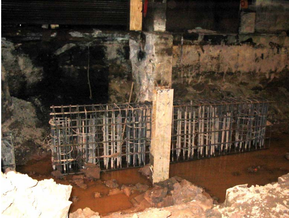
Figure 7: Cap beam reinforcing steel
