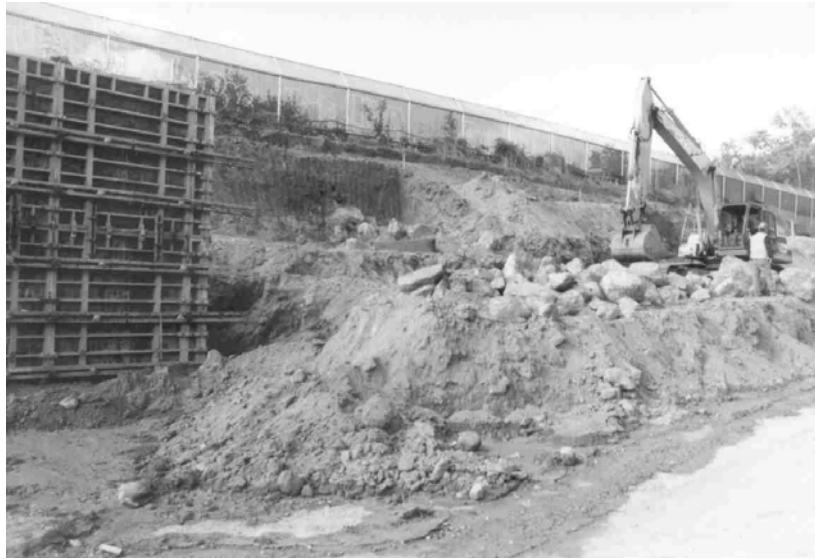
Figure 5. Excavation of Section 1.
