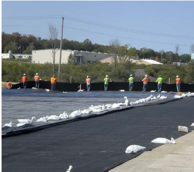
Fig. 20 Geomembrane Panel Placement
