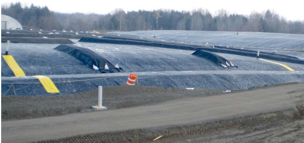
Fig. 23 Completed Cap With Sand Tubes and Access Walkways
