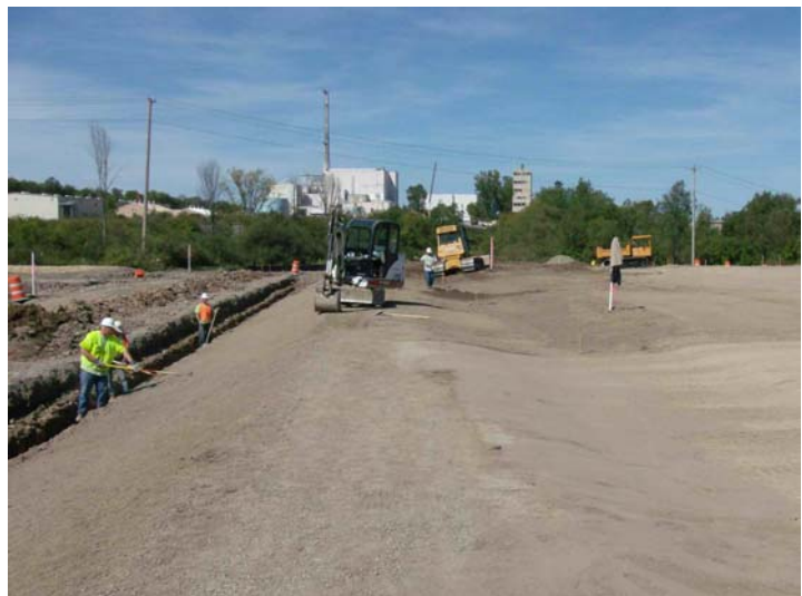
Fig. 19 Completed Barrier Wall Area
