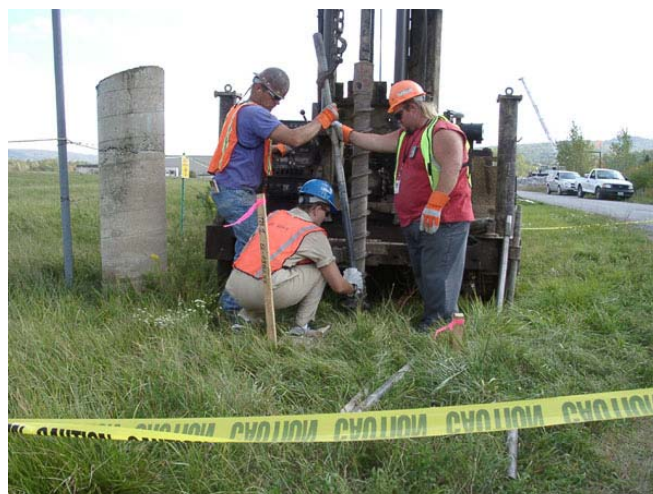
Fig. 11 Drilling Test Borings
