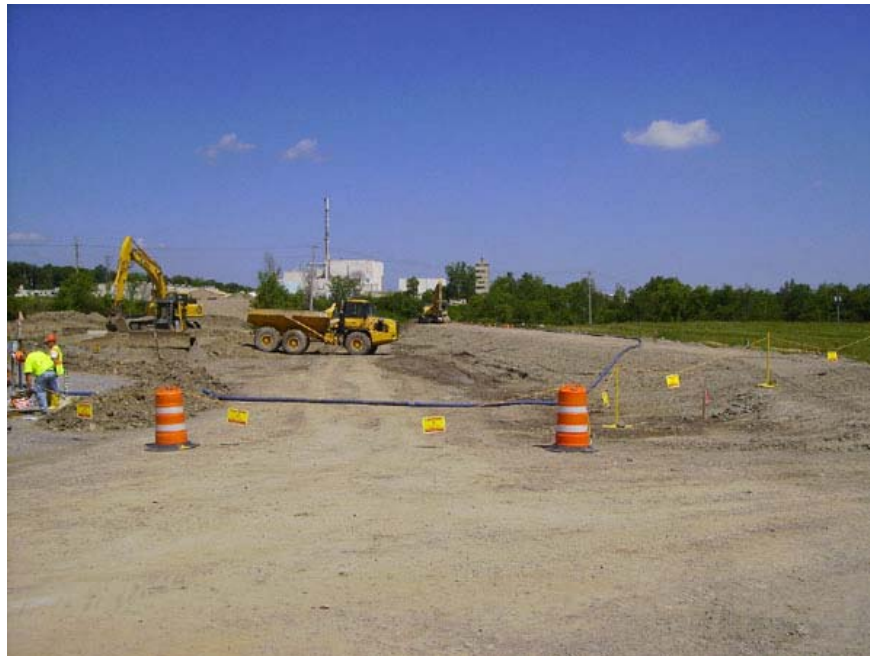
Fig. 14 Working Platform Under Construction
