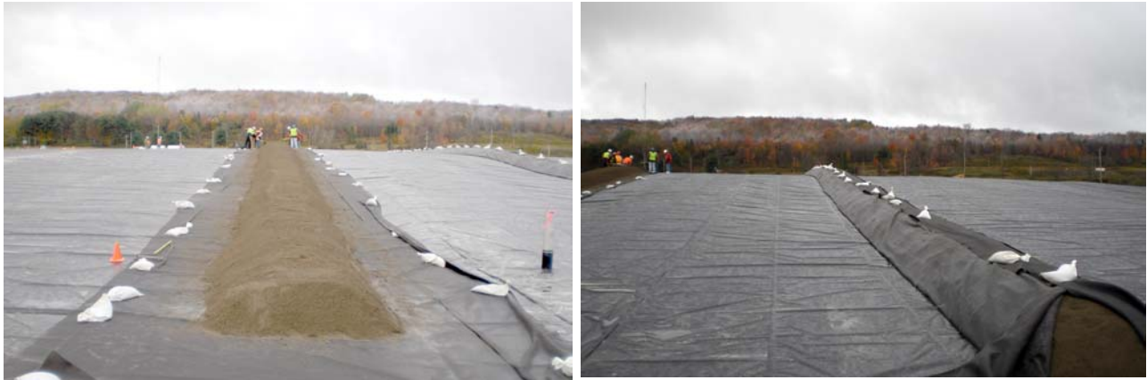
Fig. 22 Sand Tubes Placed on Geomembrane
