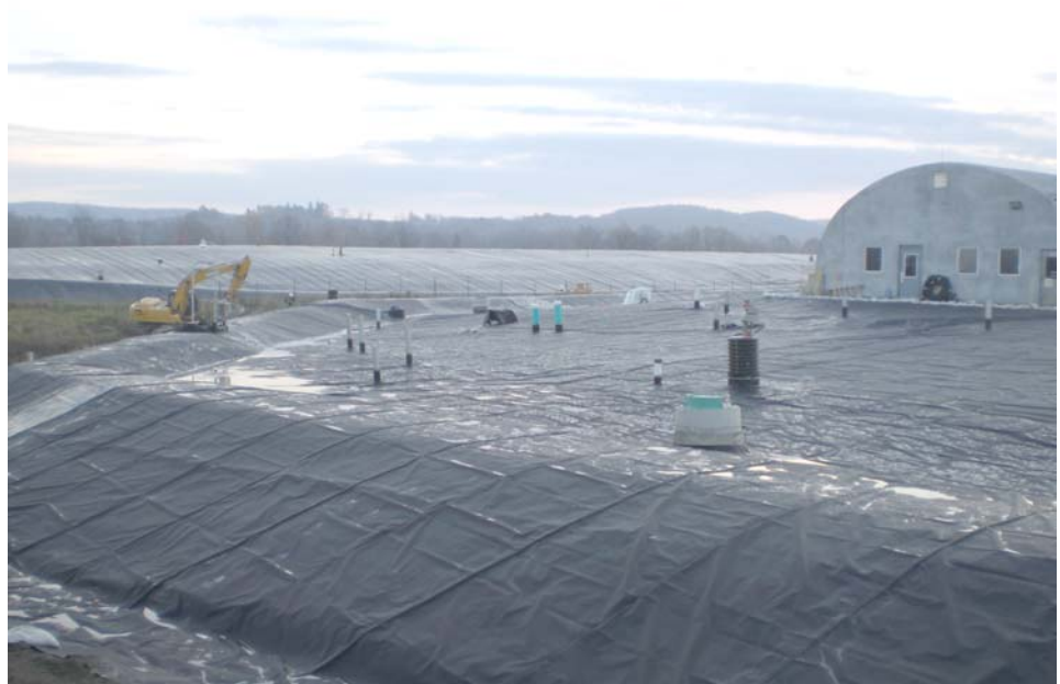
Fig. 21 Detention Basin No. 3
