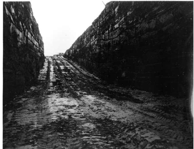
Fig. 2 Photo of Excavated Disposal Trench
