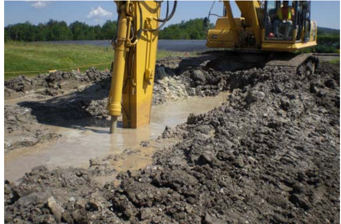
Fig. 15 Slurry Trench Excavation
