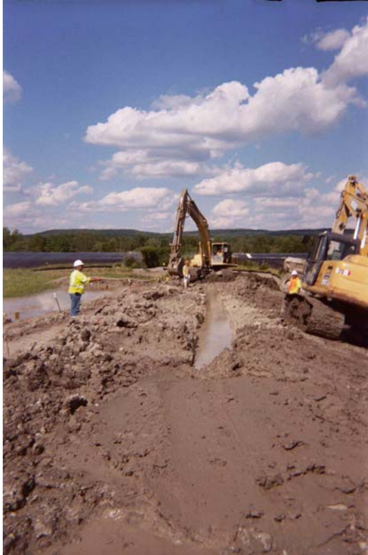
Fig. 18 Barrier Wall Excavation and Backfilling
