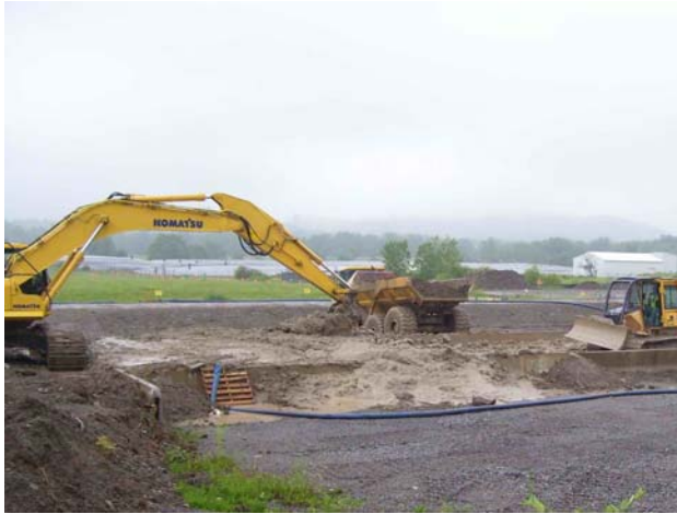
Fig. 16 Backfill Mixing Operation
