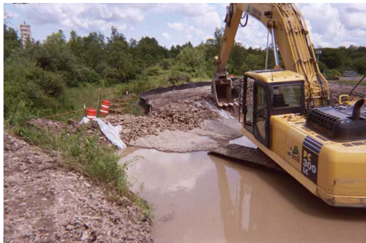
Fig. 17 Maintenance to Temporary Basin Outlet Structure
