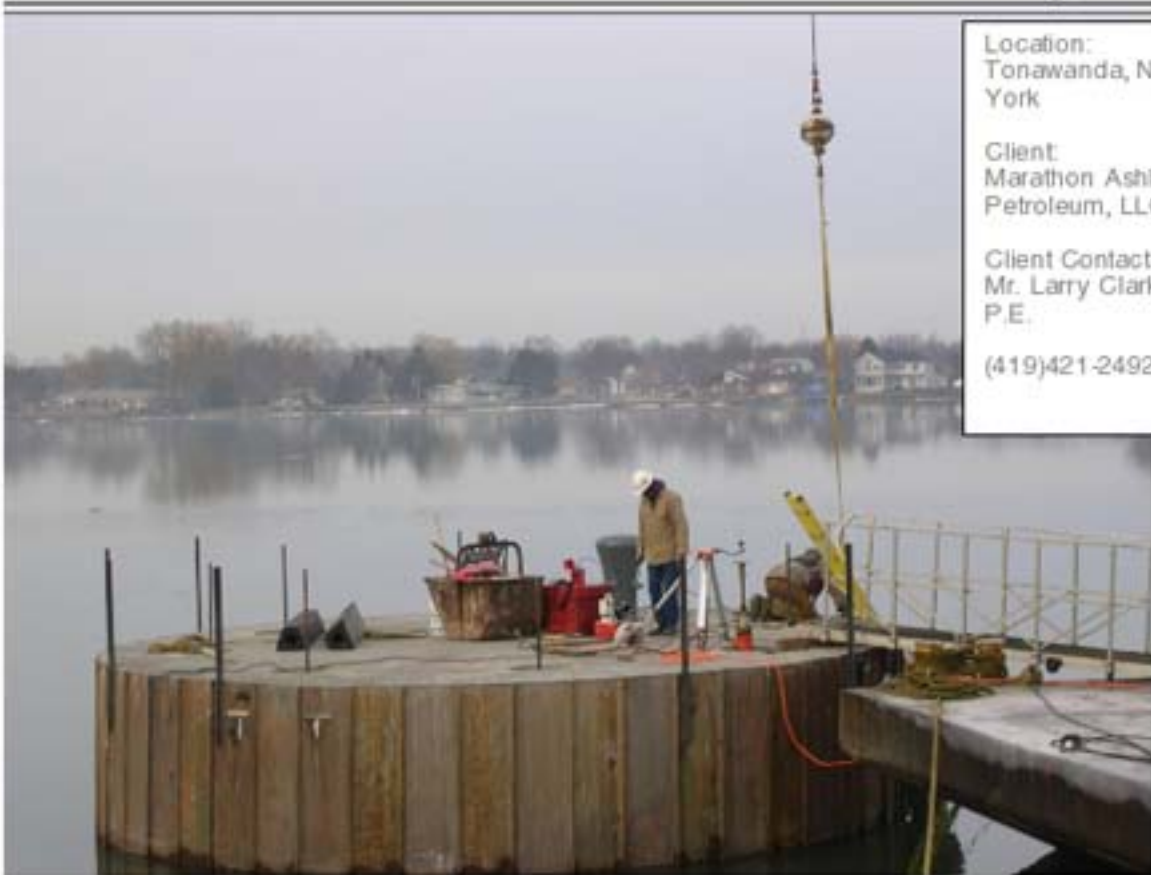
The Breasting Cell Nearing Completion in the Niagara River
