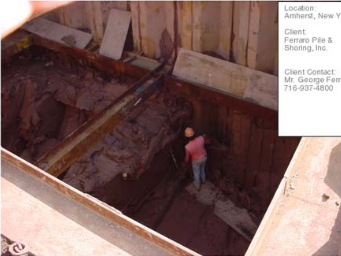
Completing the Excavation in Very Soft Clay
