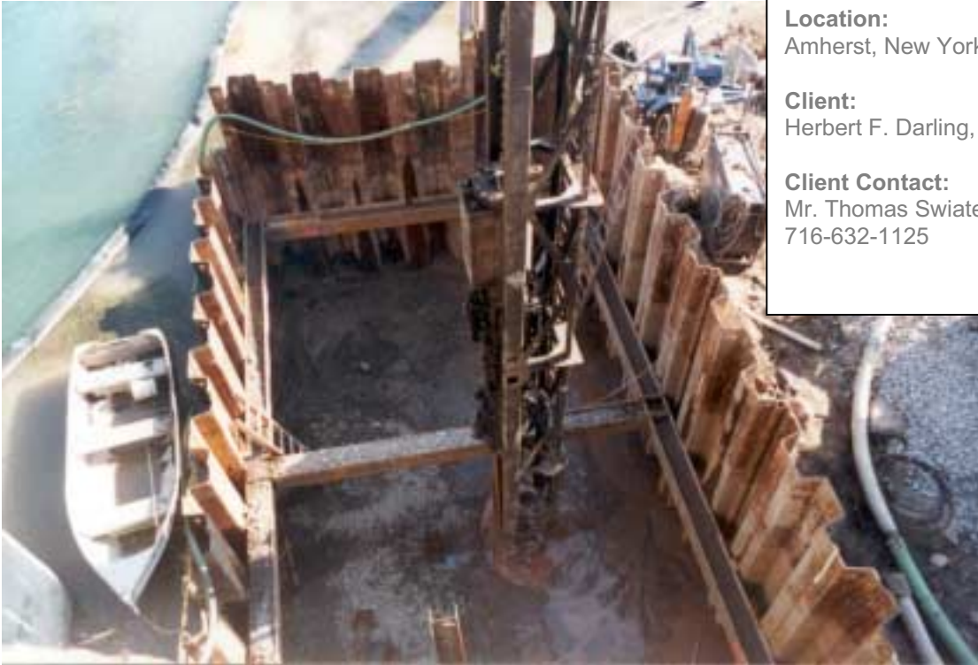
Excavation for Pier 1 during Bearing Pile Installation
