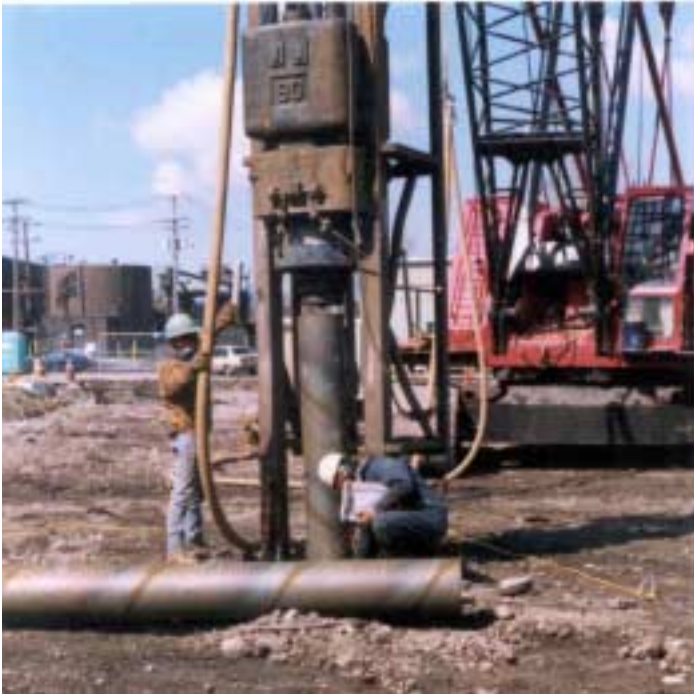
Preparing a pile for dynamic tests
