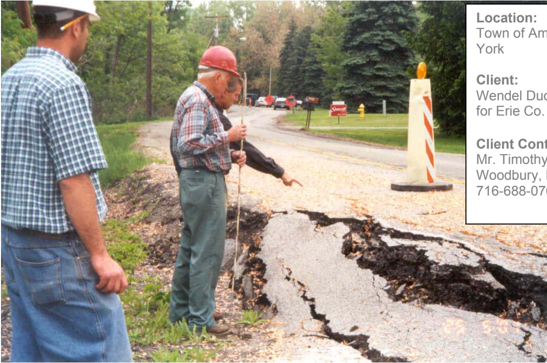
View of Slope Failure Scarp
