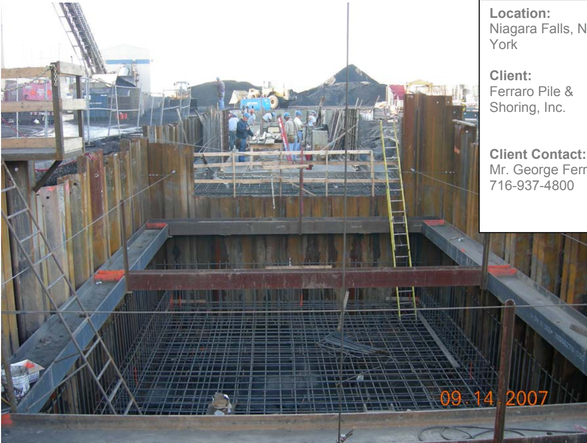
Braced Sheetpile Cofferdam with Reinforcing for the Floor in Place
