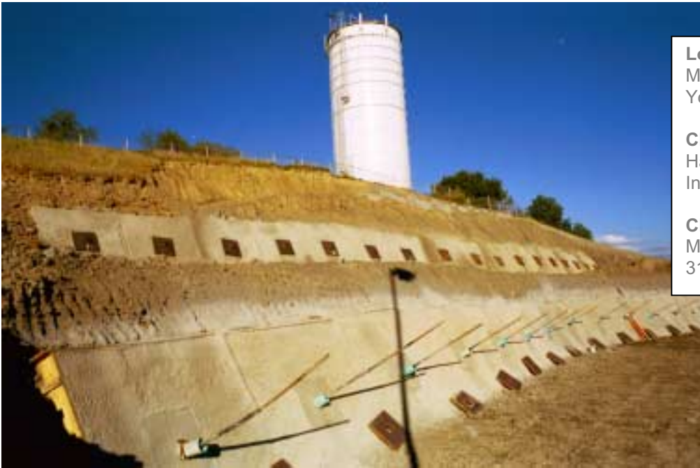
View of Reaction Block Wall
