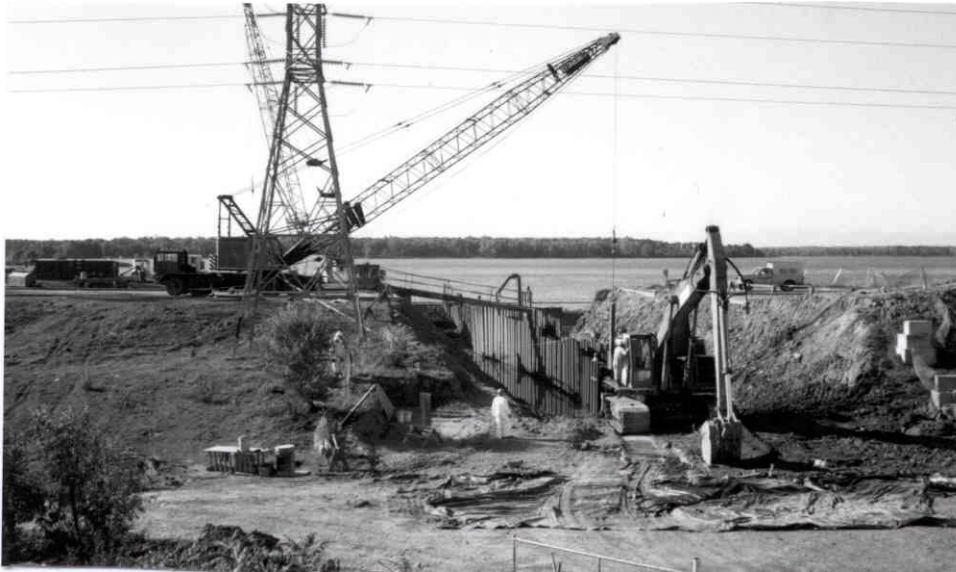
View of the Barrier Wall Construction Across the Niagara Parkway Looking South – Niagara River in Background
