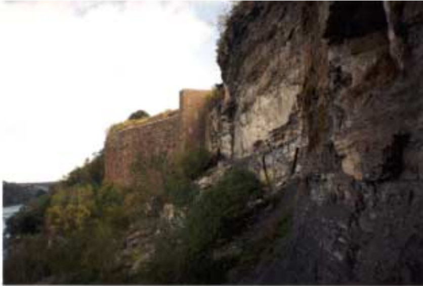
View of Schoellkopf Wall and Niagara Gorge Looking North
