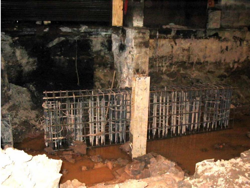
**Figure 7:** Cap beam reinforcing steel
