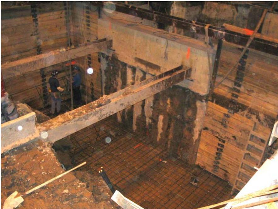
**Figure 9:** Completed secant pile wall and bracing
