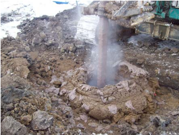
Soil Cement Column Installation
