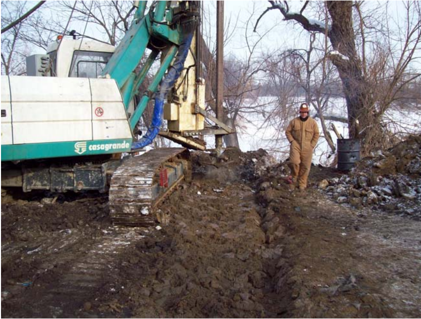
View of Dry Soil Mixing Operations
